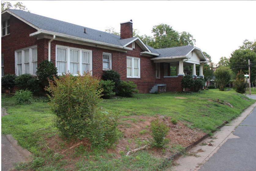
Upper End of Driveway Wall Location
